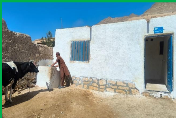
Improved Livestock Stables, Balkh Province, October 2024.
