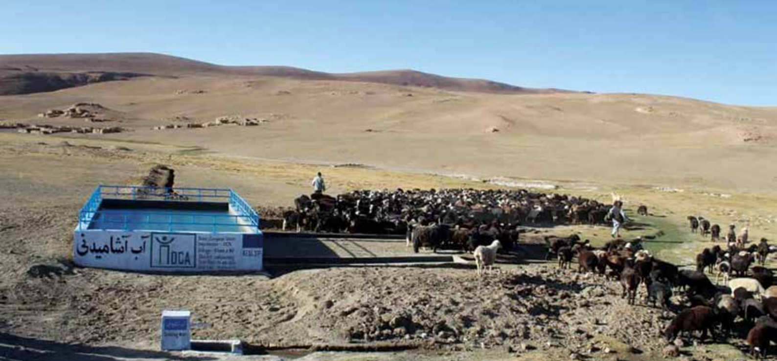
Water Reservoir, Bamyan Province
