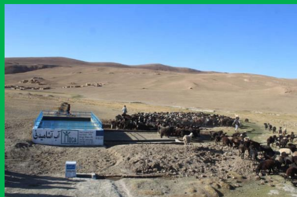
Constructed Water Reservoir, Bamyan Province, August 2024.
