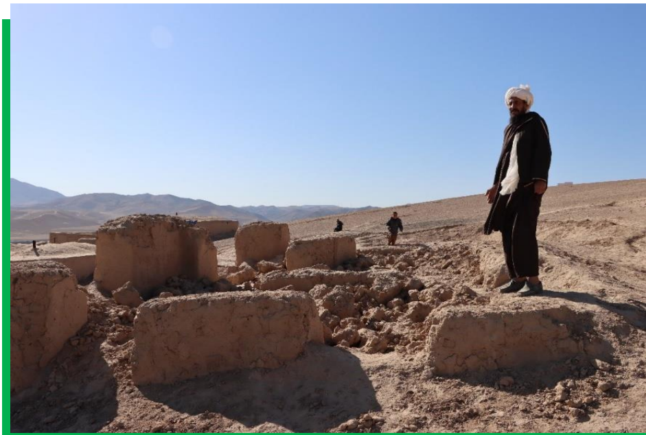
Earthquake-affected Households, Injil District, Herat Province, January 2024.
