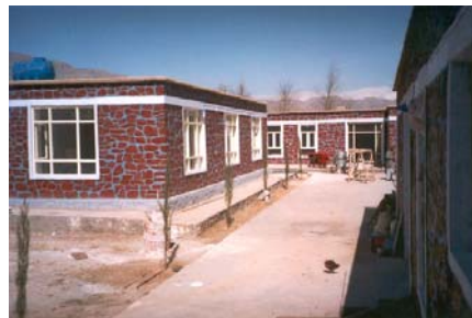
Charikar VTSC after refurbishment
